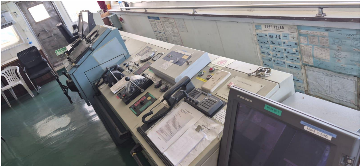
Image 9: Manoeuvring Control Console
